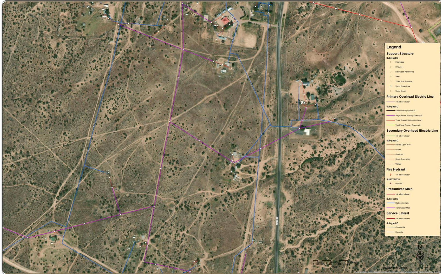
Photo 19. Central South. This photo depicts the NTUA utility infrastructure for Klageh Loop community.
